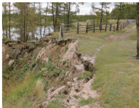
Fig.2. Destruction of roads as a result of the thawing of frozen ground. Megino-Kangalasskii ulus (district), Suola village, 2010.
