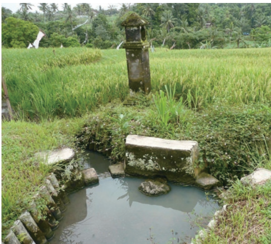
Photo 1 Diversion work in a traditional water management system 'subak' in Bali of Indonesia
