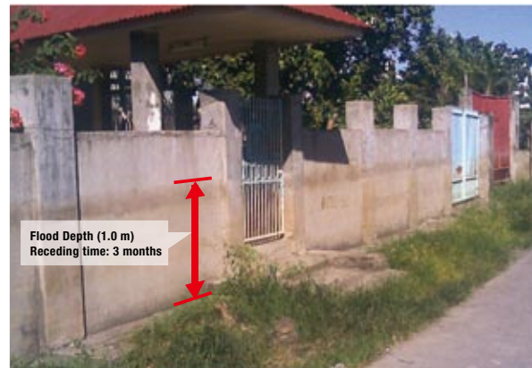
Figure 4 Extent of flood in the village of Aplaya, Santa Rosa, Laguna
