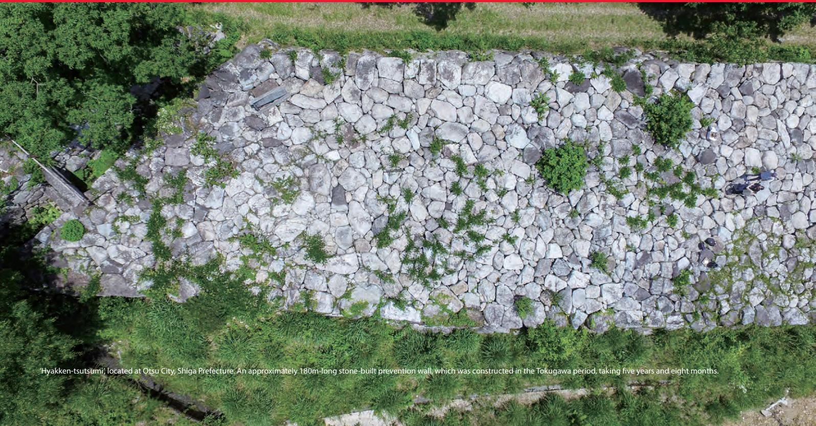
'Hyakken-tsutsumi', located at Otsu City, Shiga Prefecture. An approximately 180m-long stone-built prevention wall, which was constructed in the Tokugawa period, taking five years and eight months.
