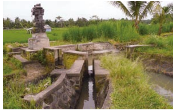
Photo 2 Diversion works of a small-scale irrigation system in Bali, Indonesia
