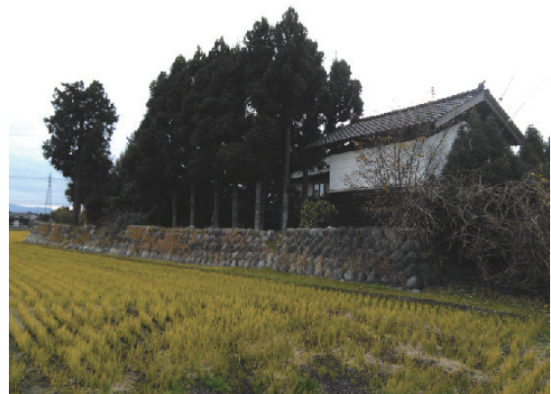
Photo 6. Big stone wall house
