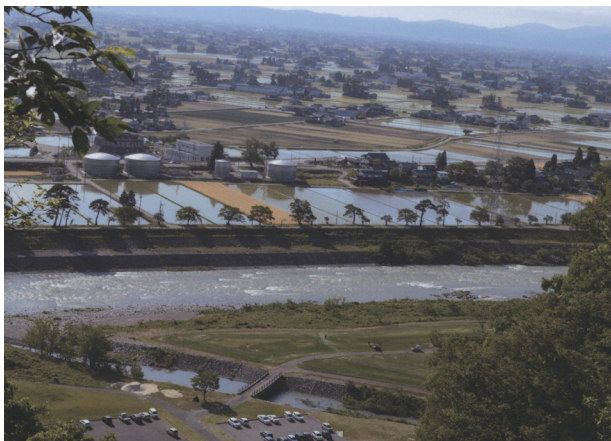
Photo 2. Pine River removal (May 23, 2021)
