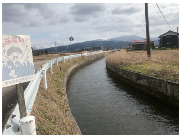
Photo 4. Well-maintained Aquaduct (February, 2020)
