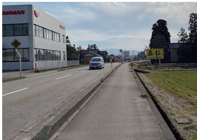
Photo 1-2. Toyama Prefectural Road No. 25 Tonami Hosoiri Line after construction (April, 2021)
