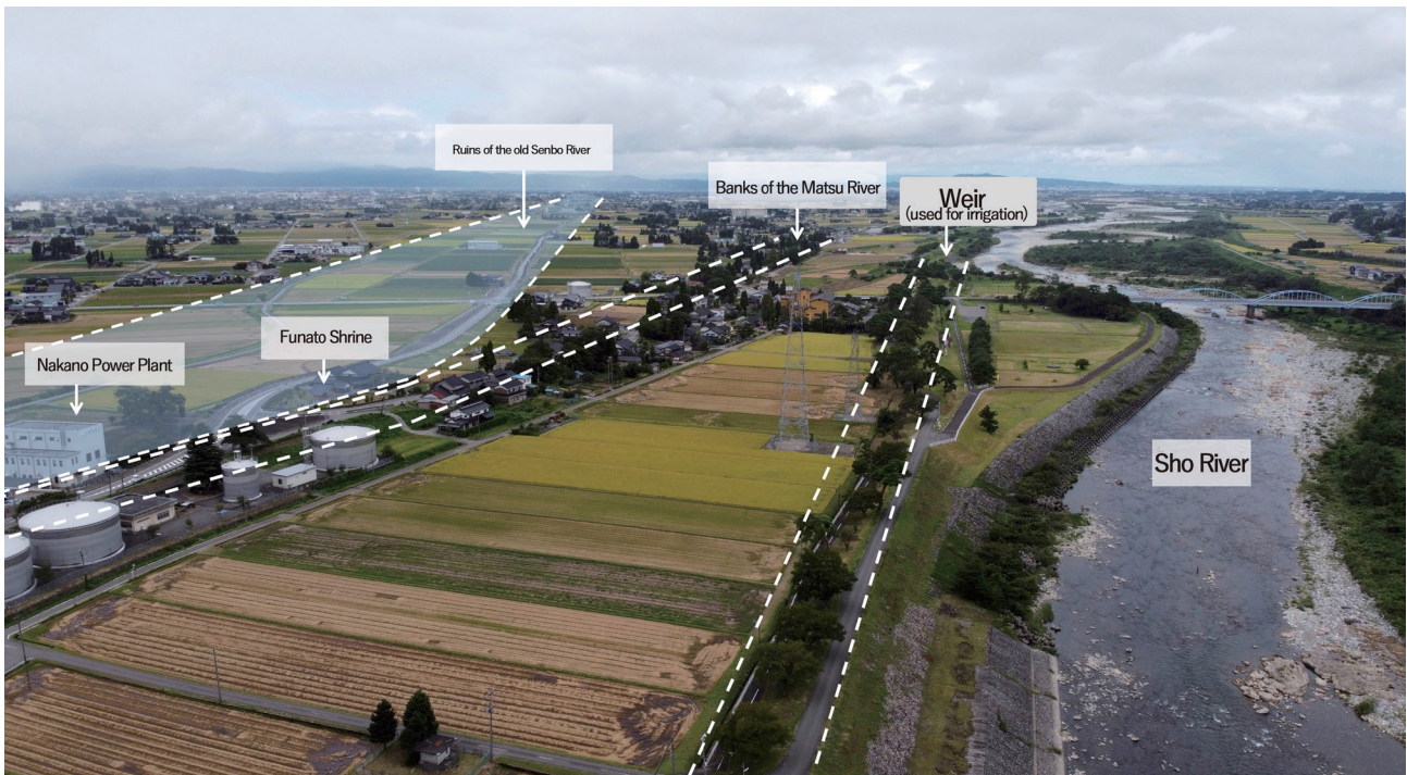
Photo 1. Pine River removal (September 14, 2020, Photo: Eco-DRR Project)
