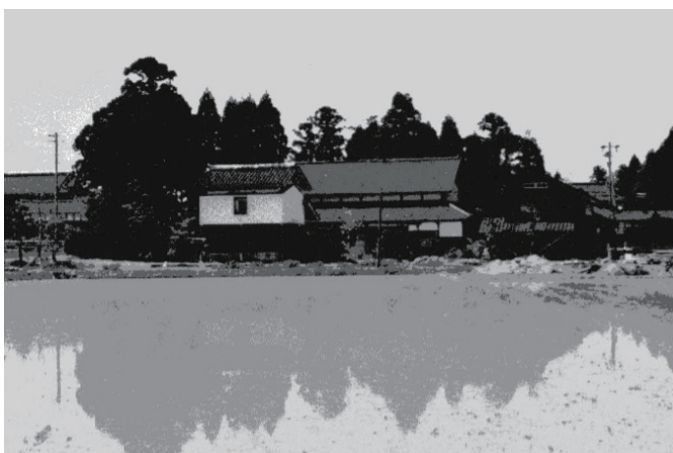
Photo 5. The NM family's house before road widening (1988 Photo: Mr. NM)
