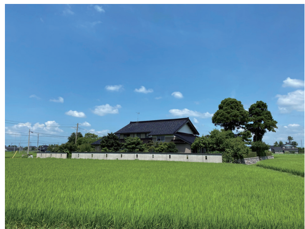
Photo 2. Exterior of Residence B taken from the southwest
