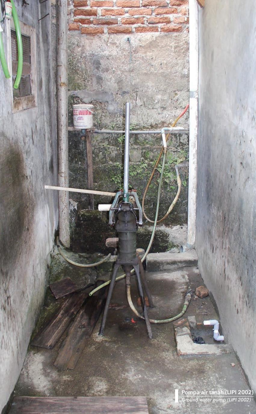
Pompa air tanah (LIPI 2002)
