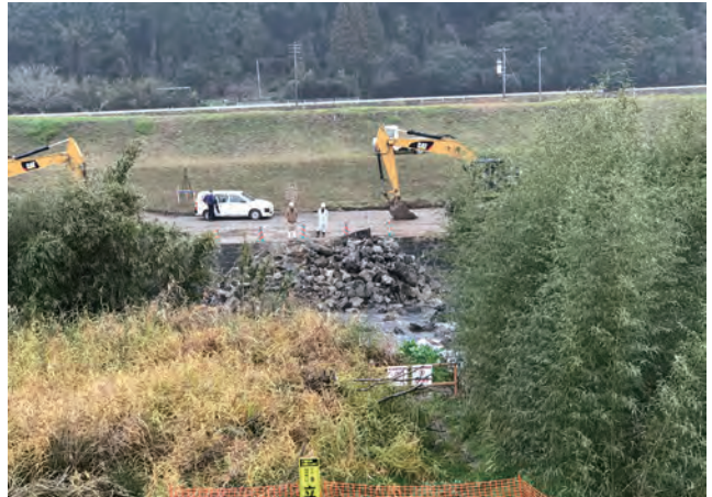
Photo 3. Removal of the Okawano flood submerging bridge
