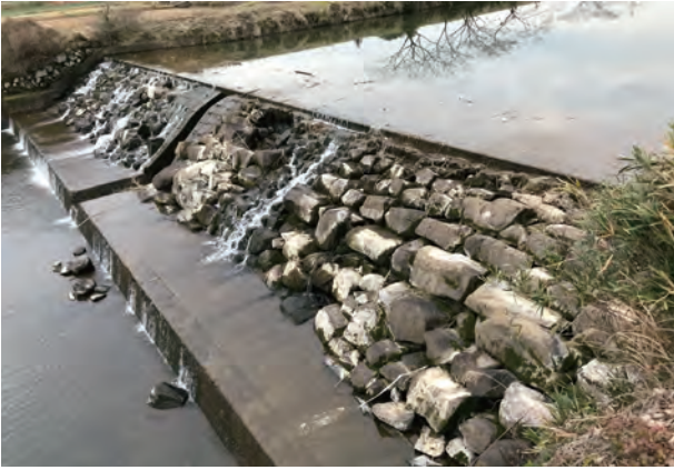
[1] A typical horizontally stacked dam
