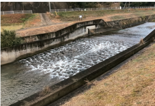
[6] A typical gentle slope dam
