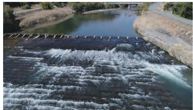
Photo 4. Kawaharazono Weir (Kanoya City, Kagoshima Prefecture)
