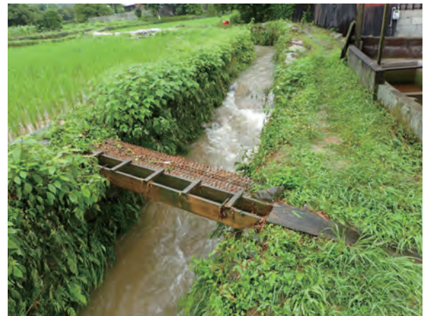
Photo 4. A wooden water pipe spanning a stream that runs around fields in Akizuki, a historic building preservation district (Asakura City, Fukuoka Prefecture)
