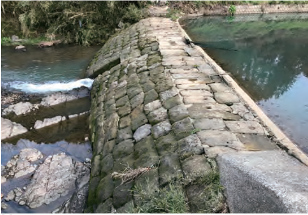
[4] A typical arch dam
