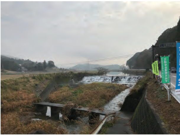
Photo 6. Flood submerging bridge downstream from a weir
