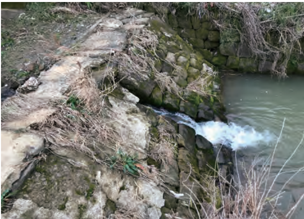
[5] A typical steep slope dam
