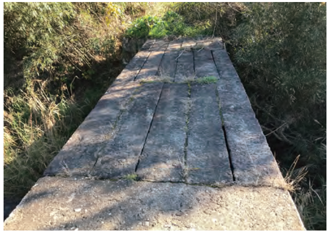
Photo 4. The Okawano flood submerging bridge had stone girders
