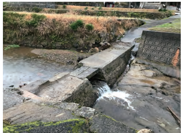
Photo 9. A low-level crossing passable only on foot
