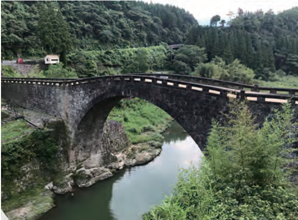
Photo 1. Reidai-kyo Bridge (Misatomachi, Kumamoto Prefecture)
