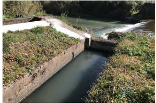
Photo 5. Umankashira outlet, divided into upper and lower channels.
