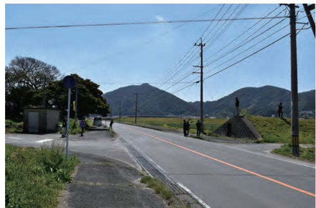
Photo 3. Floodwall gate with a prefectural road (photo: Naoto Tanaka)
