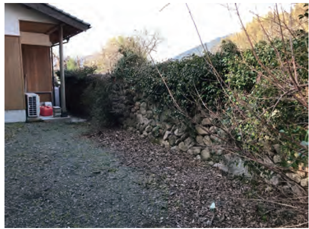
Photo 2. Stone wall surrounding a house
