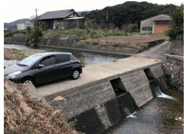
Photo 10. A low-level crossing weir passable by cars
