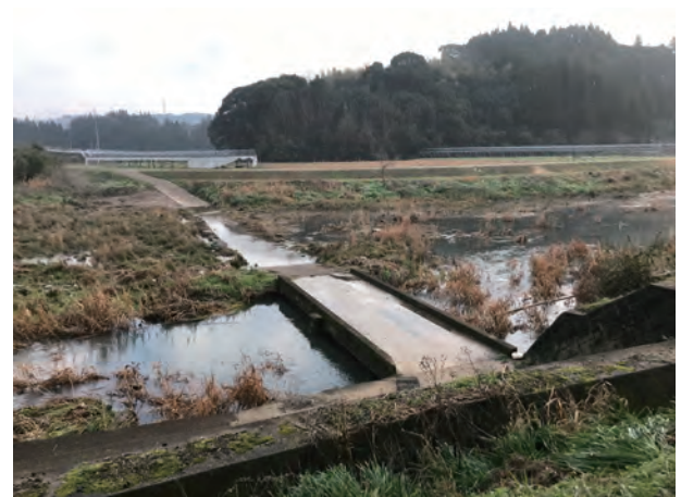
Photo 8. Flood submerging bridge and low-level crossing on the Tokusue River
