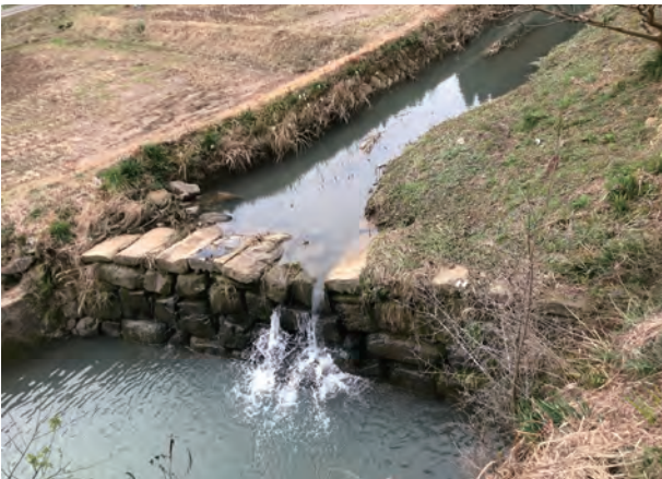
[2] A typical perpendicularly stacked dam
