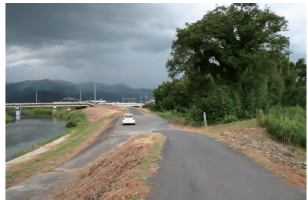
Photo 7. Jobaru River nogoshi . Part of the embankment is lowered so that flood water flows from the chosen location.
