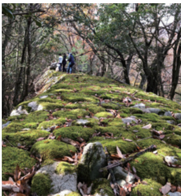
Photo 1. Stone embankment to prevent landslides
