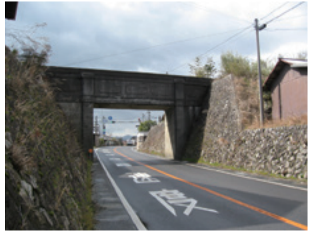
Figure 4. Raised-bed river flowing above a road, lower Yanamune River
