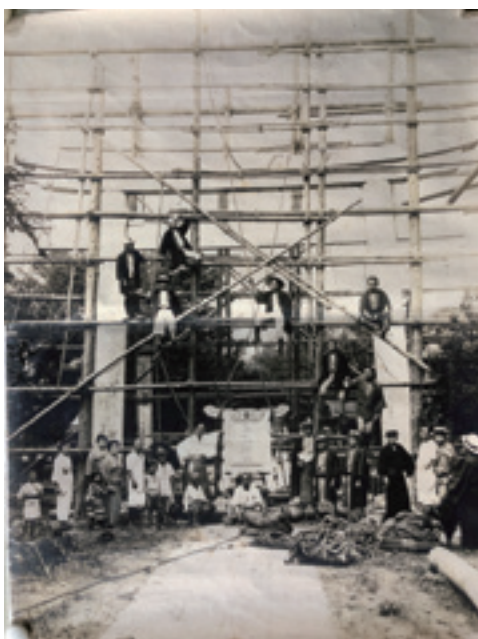
Photo 7. The state of work on construction of the Mio Shrine tori-gate
