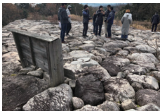
Photo 8. Hyakken (100-ken) Embankment
