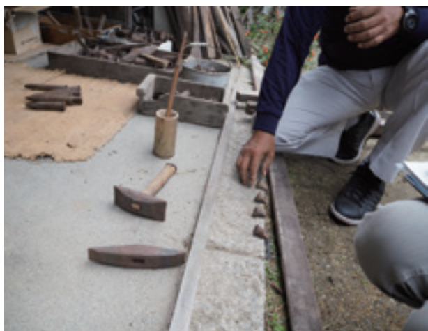
Explaining how to split stone using a real curbstone (November 21, 2016).
