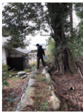
Photo 7. Stone embankment near Hachiman Shrine
