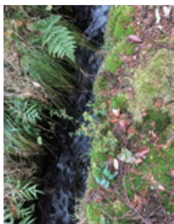
Photo 4. Water supply aqueduct in Moriyama
