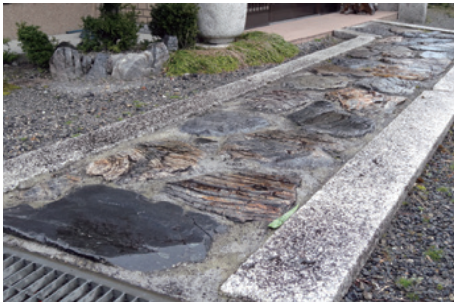
Photo 2. At a private residence at the foot of Mt. Hira. Local stones have been used in the approach to the entrance. The white stone used at the edges is granite, and the striped stone is bedded chert.
