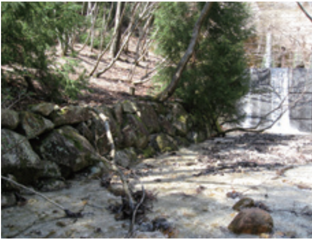
Figure 3. Stone embankment ruins and erosion control dam in the upper Yanamune River
