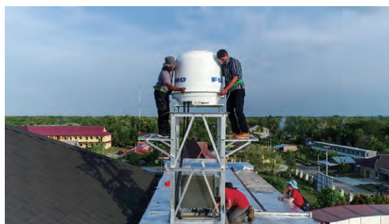
Weather radar installation (Bengkalis District, 12 February 2020)
