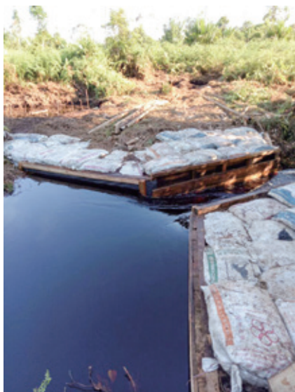
Photo 1 Rewetting by small wooden dam in Kepau Baru village, Meranti, Riau
