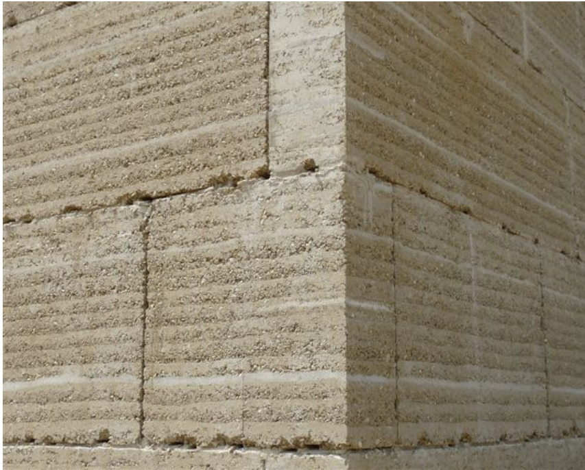
Prefabricated Elements, Ricola Herbal Center 2013
