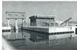
Flood control gates 25
