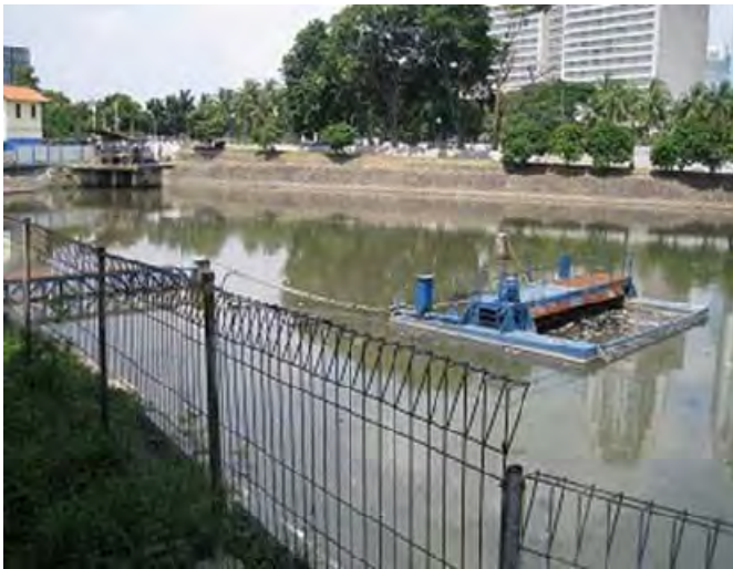
Pic.4 Sewage plant of PD PAL JAYA
