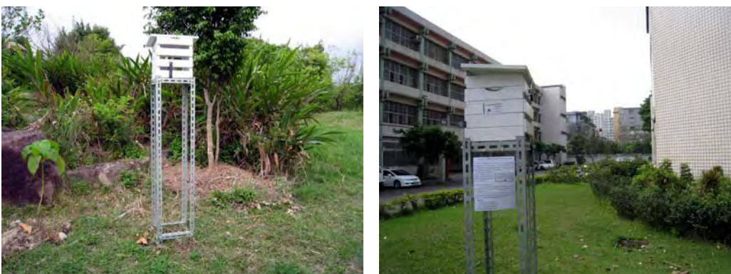
Fig. 7 Thermal recorder installation
