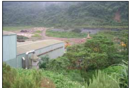
Fig. 8. Nankang Landfill facilities in Taipei.
