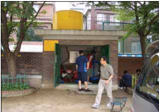
Fig. 1. Groundwater observation well for emergency
