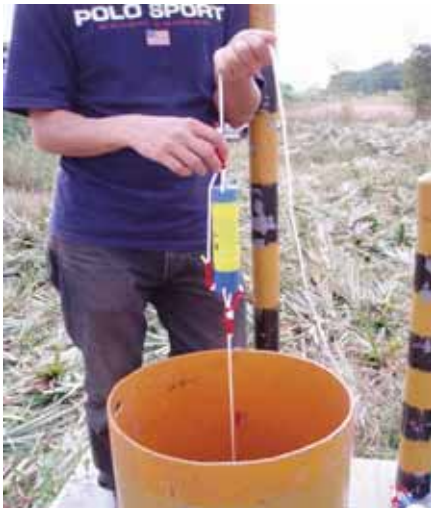
Fig.3. Installation of water temperature recorders in a borehole in Tungkang area.
