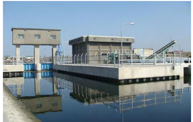
Flood control gates
