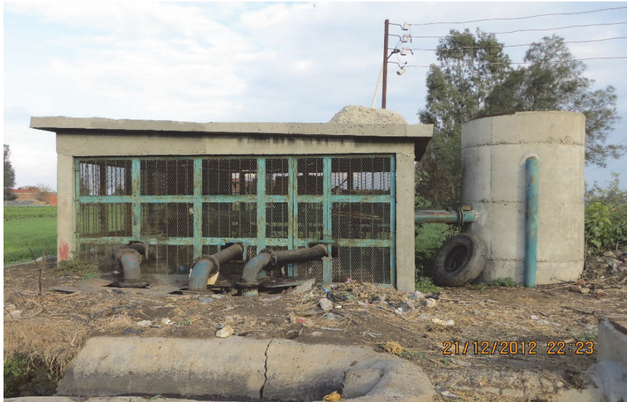
Edrega Pump Station
