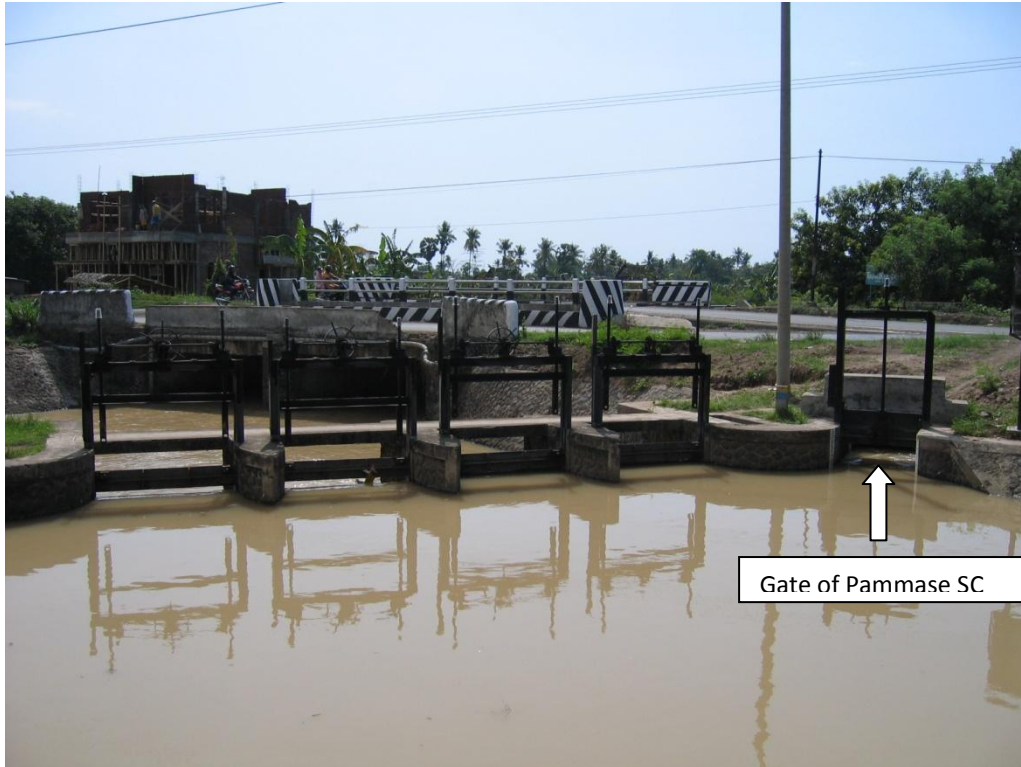
Figure 2. Gate of Pammase secondary channel at BL17 point on Kampili Primary Channel
