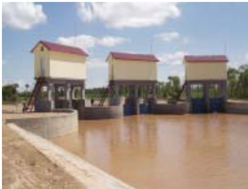
Photo 2 Water gate on Yongji Main Canal from which Xile Secondary Canal takes off
