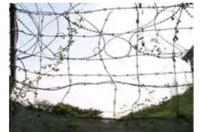
Photo A barbed-wire fence that divides a military base and local society
