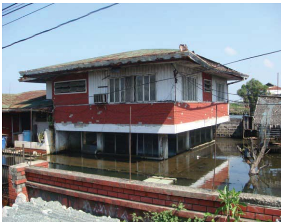
Figure 2. An abandoned house after heavy flooding
