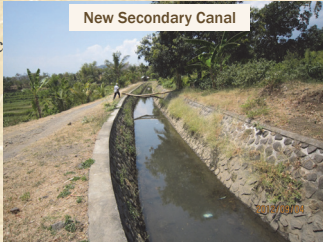
New Secondary Canal
