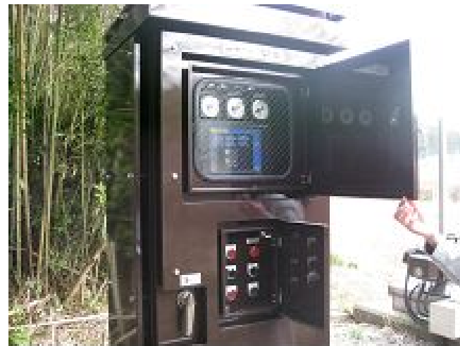
Automated water intake gate and water level monitoring
