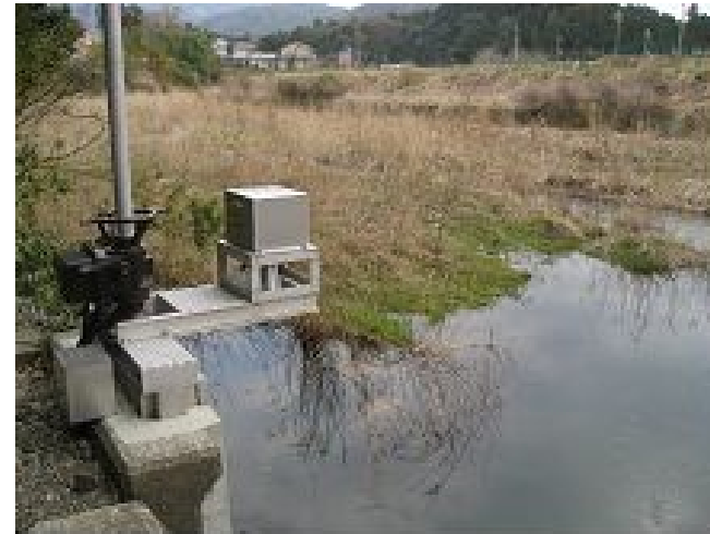
Automated water intake gate and water level monitoring
