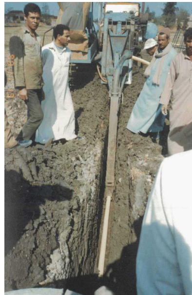
Sub-surface drain
