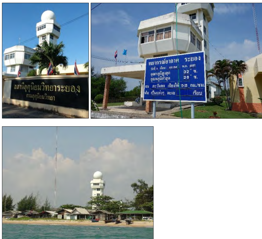
Fig. 1-2 Thai Meteorological Department in Rayong.
